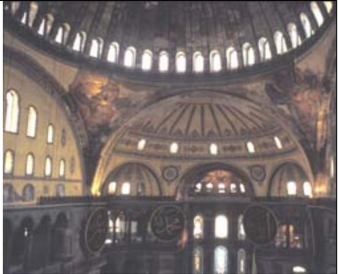
Fig. 12 – The dome, the pendentives and the arches which support the dome
