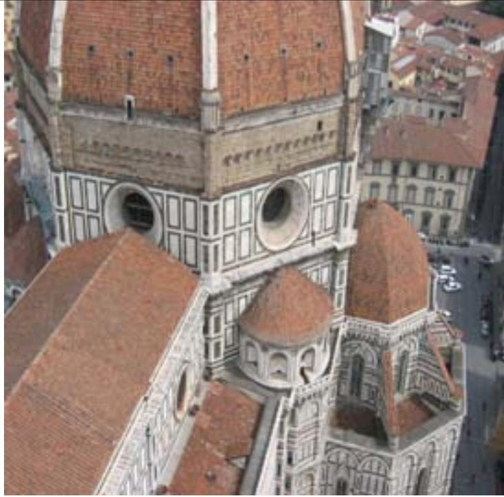
Fig. 9 – Small hemidomes which stabilise the structure of *St. Mary*
