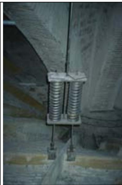
Figure 41: The tie bars and springs which connect the ribs to the roof
