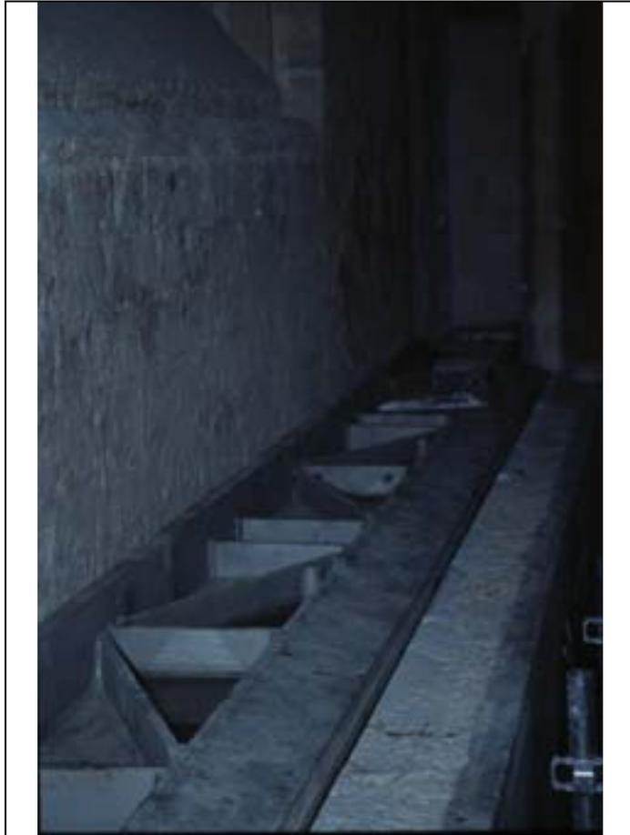
Figure 42 : The trussed steel beams placed over the cornice
