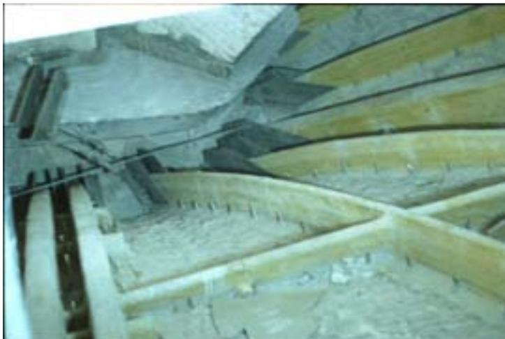
Figure 40: The ribs covered with aramidic fiber tissue
