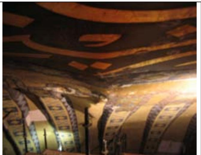
Fig. 16 – One of the discontinuity lines in the junctions between the original and rebuilt portions of the dome
