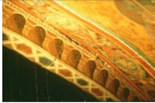
Figure 31: Cracks and detachment between webs and ribs
