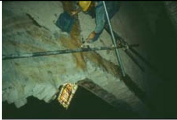
Figure 33: Little synthetic fiber strips applied over the vaults
