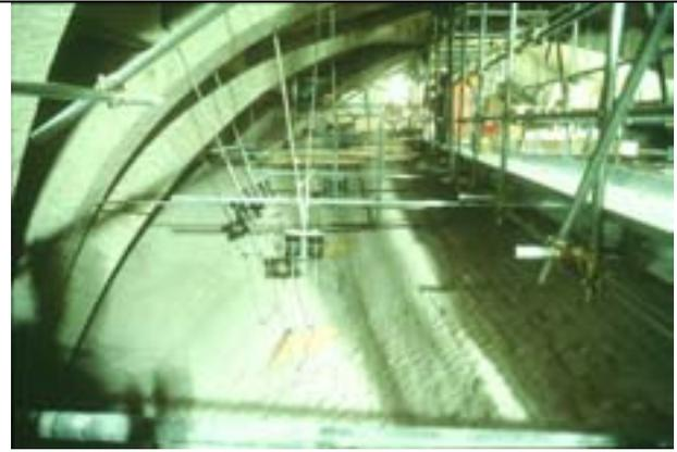
Figure 34: The system of wires and springs to suspend the vaults to the roof
