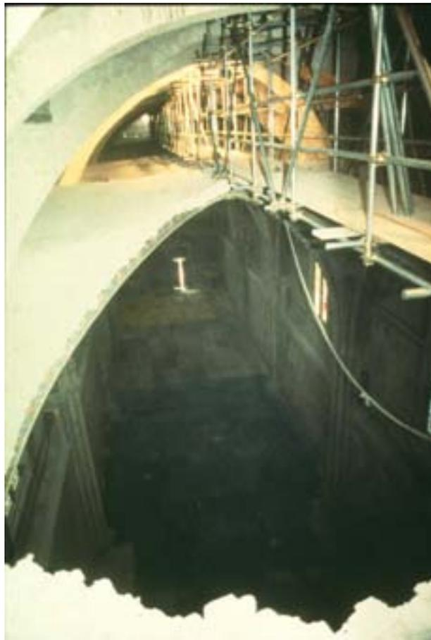
Figure 32 : The little flying bridge suspended to the roof to inspect and strengthen the vaults
