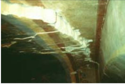
Figure 30: Large cracks with relative movements of around 25 cm
